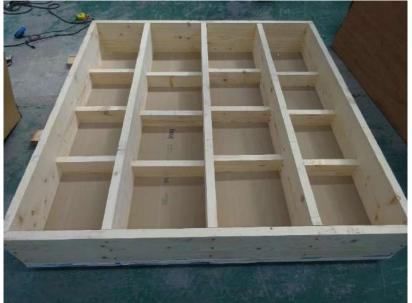
Photo No. 5 **Ceiling Assembly Being Constructed**
